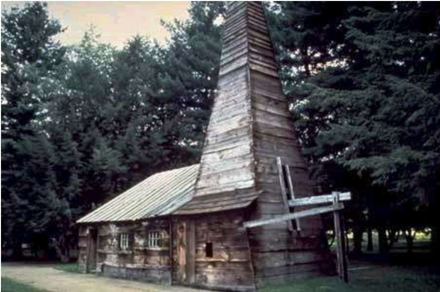
Figure: (1-1) first old rig
