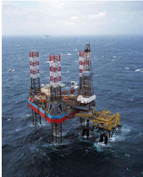
Figure: (1-5) Bottom-Supported rigs
